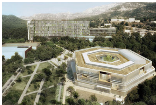
Fig. 5: Architect's view after restoration. © Rémy Marciano.
