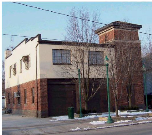
Fig. 3: View of Fire Hall No. 6 before renovations. © City of Windsor, Nancy Morand.
