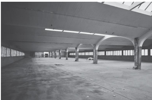
Fig. 6: The upper floor before reconstruction. © Michael B. Frank.
