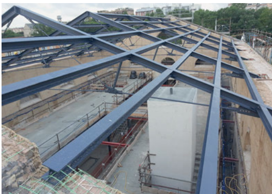
Fig. 8: First phase of the working process for the roof construction, made of steel structures. © Cesare Feiffer.
