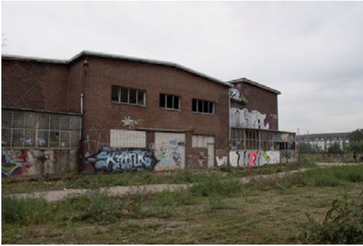
Fig. 2: Exterior before restoration. © Robert Niess.
