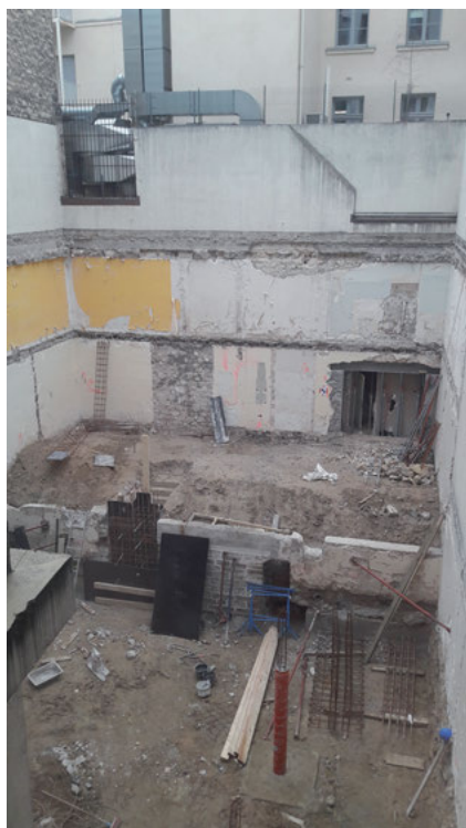
Fig. 2: Demolition of the old courtyard. © AUP.
