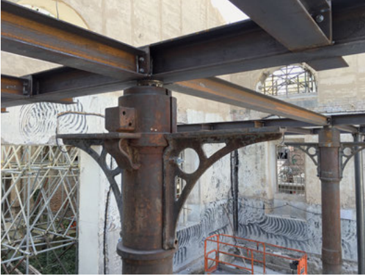
Fig. 11: Structure of the industrial archaeological elements are used as new structural elements for the new mezzanine. © Cesare Feiffer.
