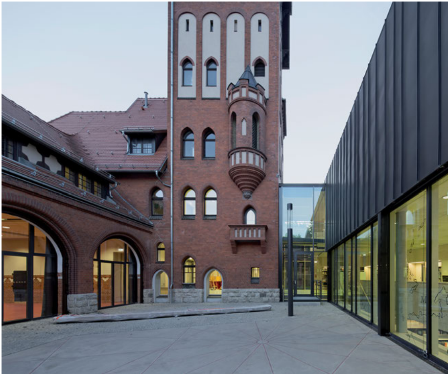
Fig. 10: The library's courtyard with the former hose drying tower and its false architectural elements used for fire brigade practice. © Werner Huthmacher.
