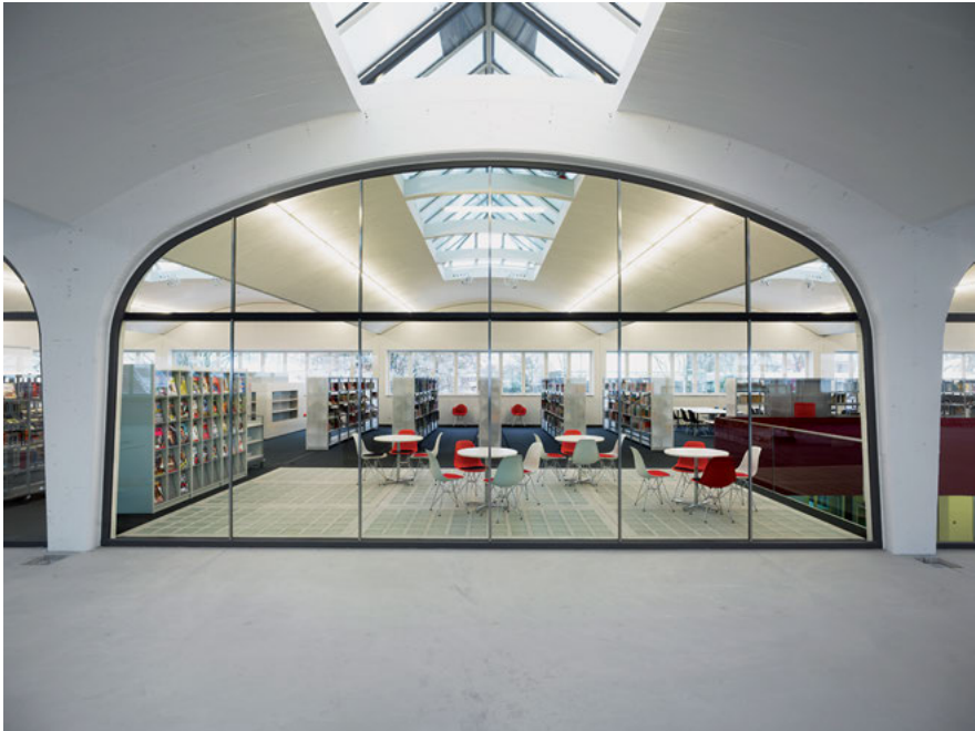
Fig. 14: The library: the fitted glass walls allow a functional division of the old production hall without destroying the spatial context. © Wolfram Janzer.
