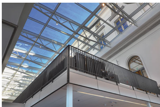
Fig. 8: The glass roof and the atrium in which a floating platform was placed. © Hilde Christiaens.
