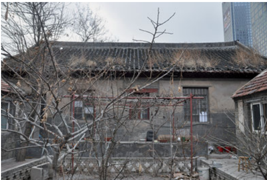
Fig. 3: Inside the courtyard before the renovation. © Suochengli Neighbourhood Library.
