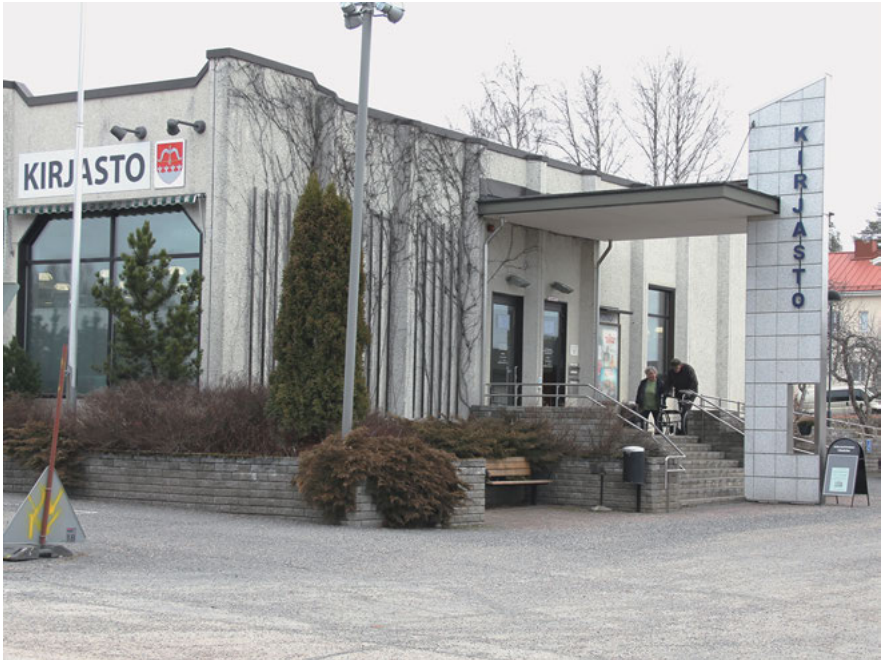
Fig. 1: The Joutsa Public Library moved into a renovated former grocery store from the late 1970s. © Eero Peltoniemi.
