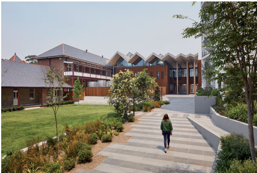
Fig. 8: Northern view from Hospital Lane. © Tom Roe.
